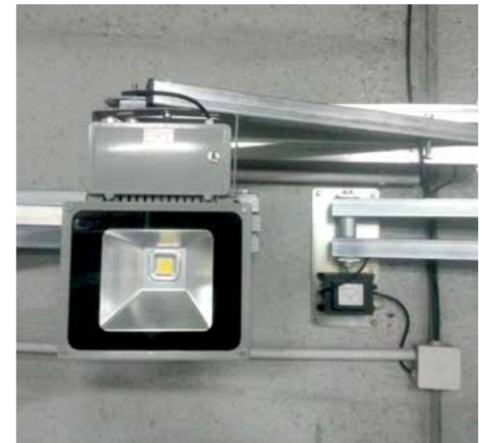
Dock light. The dock light is the perfect accessory to illuminate the interior of the trucks during loading and unloading operations.
