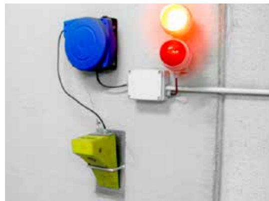
Manual wheel chock with sensor
